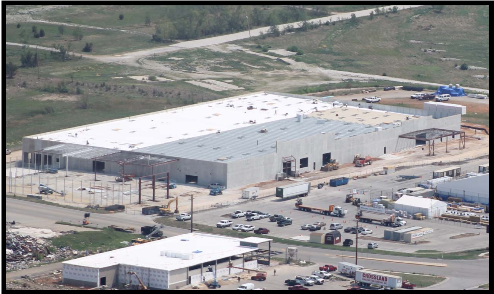
Aerial Progress Photo 8/19/2011
