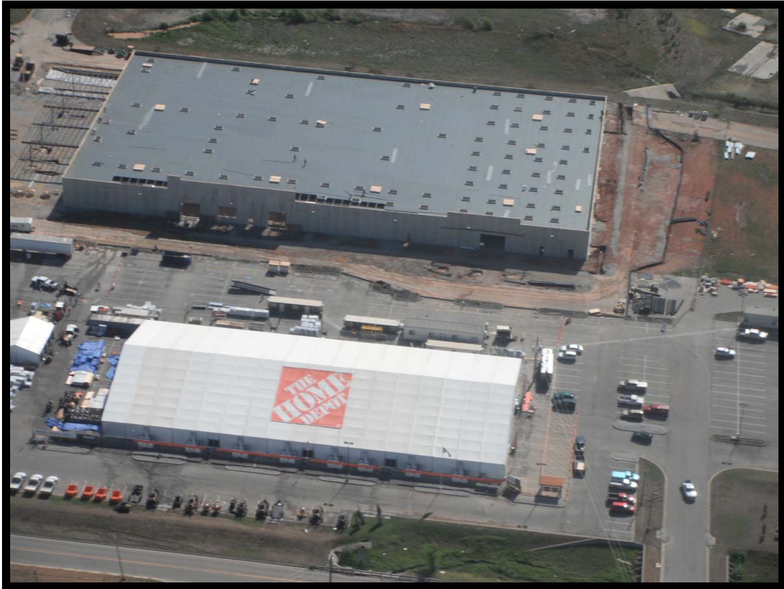
Aerial Progress Photo 8/13/2011
