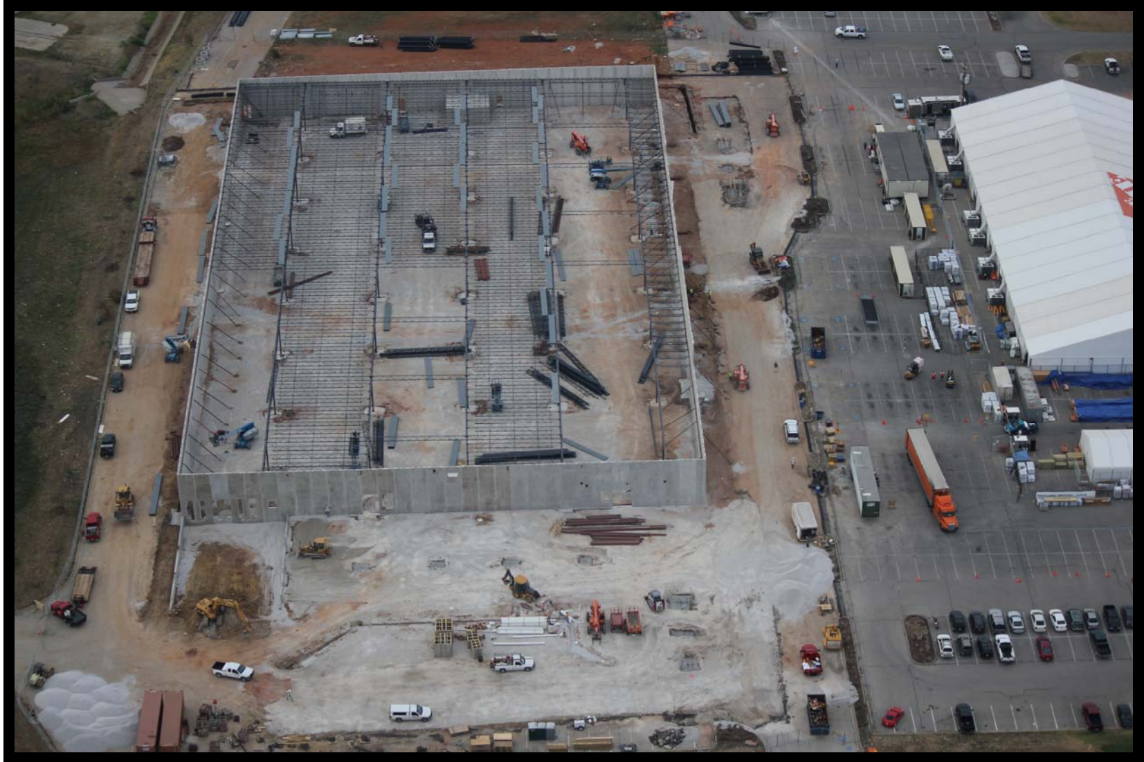
Aerial Progress Photo 8/5/2011
