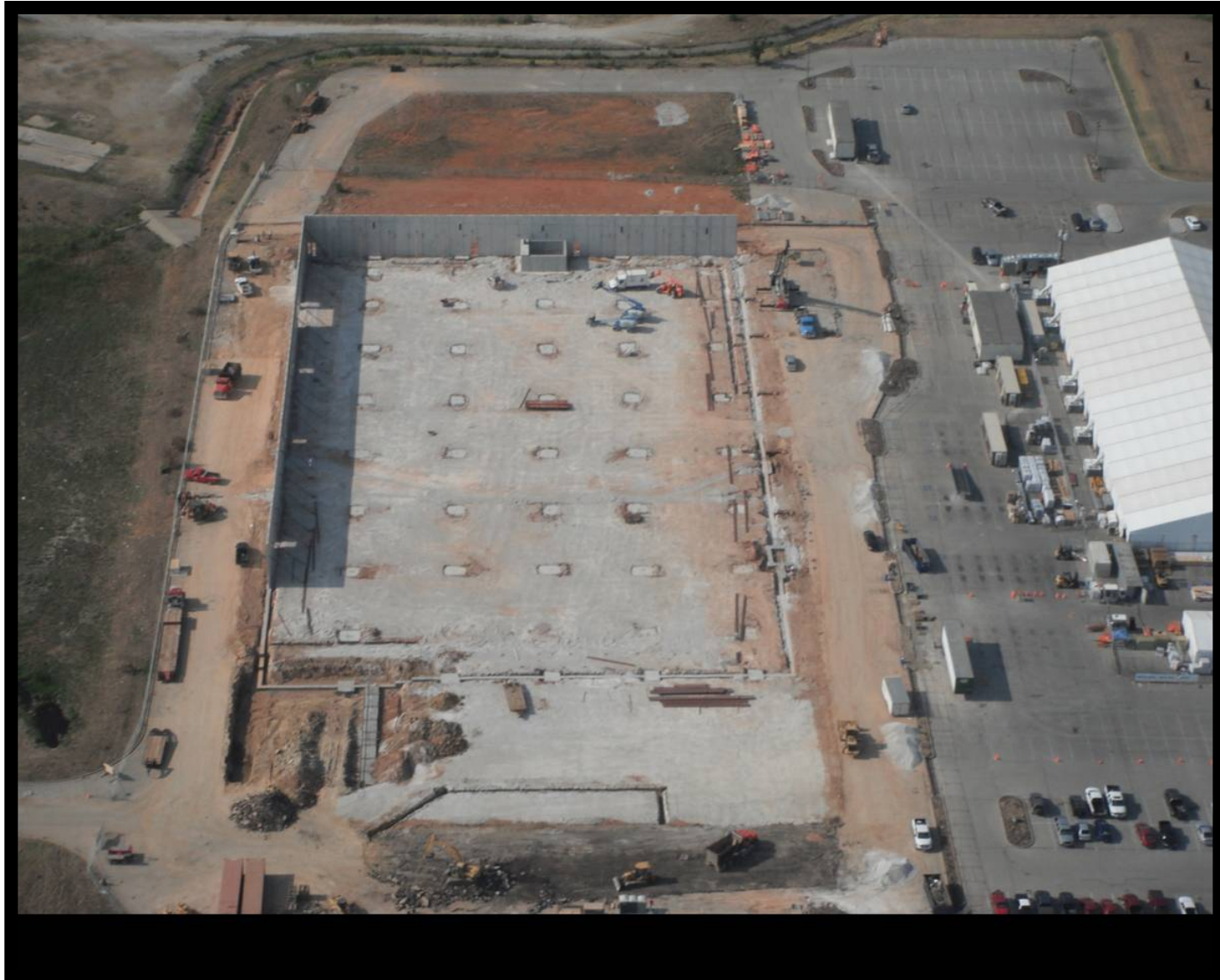
Aerial Progress Photo 7/29/2011
